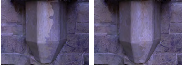
Figure 4. Pre-processing keyframes: (left) without gain compensation; (right) with gain compensation.
