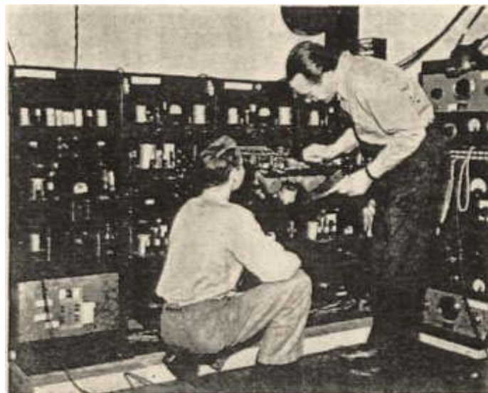
FIG. 15. View of part of the dubbing monitoring equipment. (Messrs. Hawkins and Garity.)
